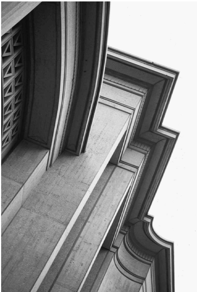
2. Corner detail, Musée des Travaux Publics, 1937. Courtesy of Brigitte Desrochers.
